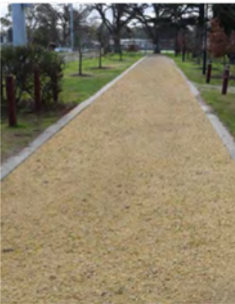
Asphalt surface with a granitic sand topcoat and concrete edge strips
