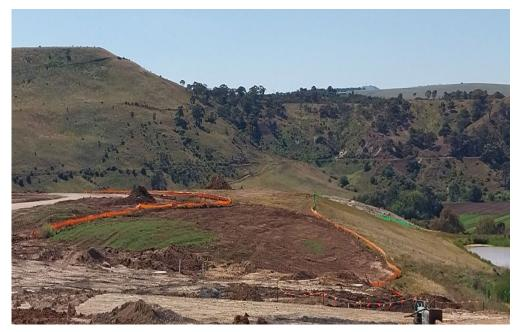
Figure 5 – Silt fencing for sediment control
