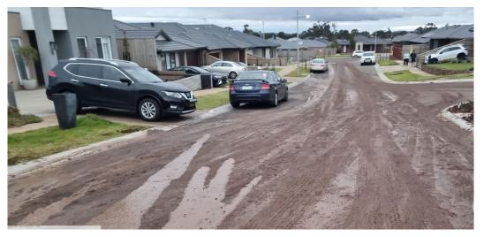
Figure 3 – Mud on Road washed to the underground drainage system.
