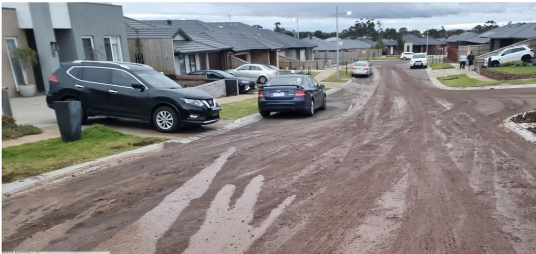
**Figure 3 – Mud on Road washed to the underground drainage system.**
