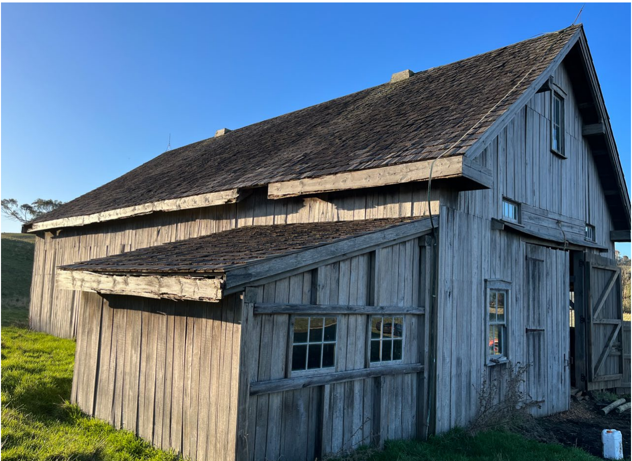
Figure 3: Photo of the Arable barn in its current condition.
