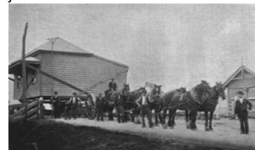
Figure 6.71: Dwelling being relocated across narrow gates of Buninyong Railway line by J.M. Williams, House Remover, c.1900. Source: Ballarat & District in 1901, plate 213.
