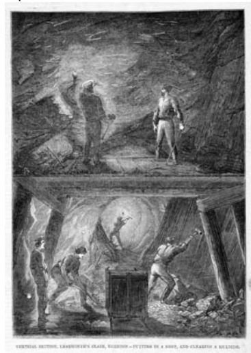
Figure 4.38: Learmonth's Claim, section drawing showing putting in a shot & clearing a reading, Illustrated Australian News , 1869. Source: La Trobe Picture Collection, State Library of Victoria, image mp001536.
