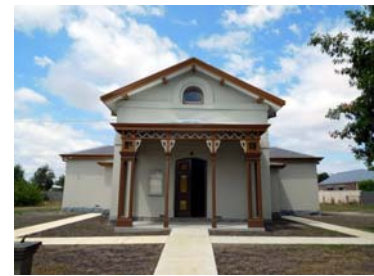
Figure 7.19: Ballan Court House, 201065, following repairs & showing reconstructed timber verandah (based on design of 1874-75). Source: David Rowe.
