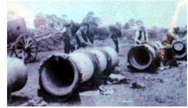
Figure 4.49: Transportation of recently-constructed concrete pipes, Wallace, c.1910. Source: Brazenor & Odlure, History of the Ballarat Water Supply .
