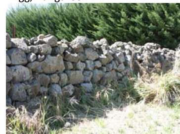
Figure 4.32: Detail of Dry Stone Wall, Clarendon, 2009. Source: David Rowe.
