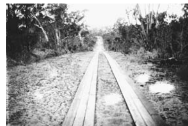
Figure 3.08: Plank Road near Osborne Park and Scarborough, Western Australia, 1911-19. Similar plank roads were established at Clarendon. Source: State Library of Western Australia, image 011296d.
