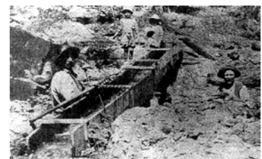
Figure 4.34: Sluicing at the Blackwood goldfields, n.d. Source: Buckingham & Hitchcock, Aspects of Early Blackwood , p.16.
