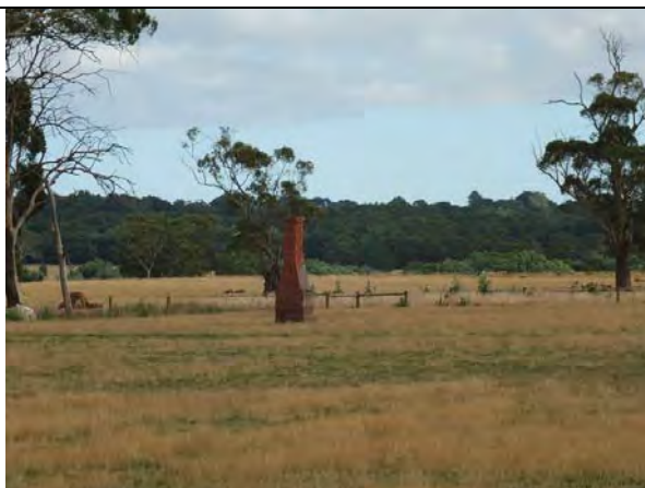
Photo 4: Surviving chimney stack from an earlier building, south-east of the elongated gabled outbuilding, 2015.
