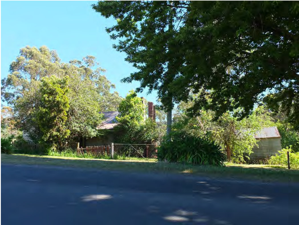
Photo 2: Dwelling, 58 Main Street, with outbuilding on the right, 2014.
