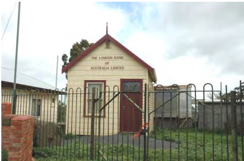
Photo 2: Former London Chartered Bank of Australia Limited, Bungaree, 2009.
