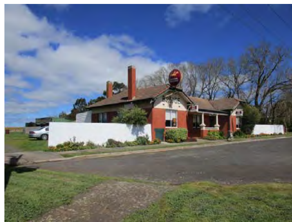
Photo 4: Bridge Hotel showing front & east elevations, 2016.
