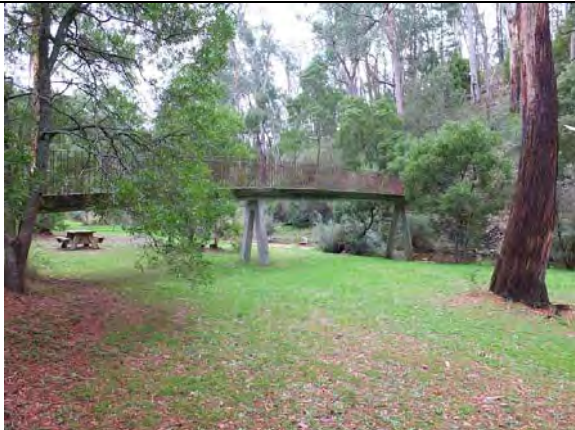
Photo 5: Concrete bridge spanning the Lerderderg River, 2014.
