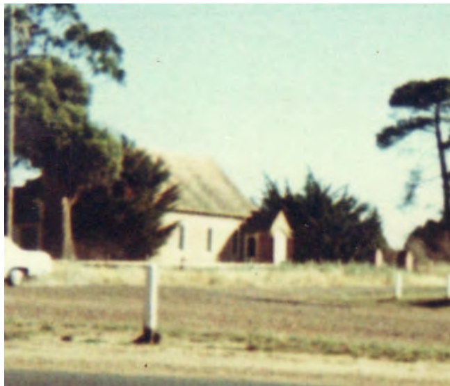
Figure 4: St Mark's Church of England Church, Gordon, c.1967.
