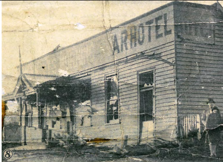
Figure 3: Substantially damaged Morning Star Hotel caused by the cyclone, 1927.
