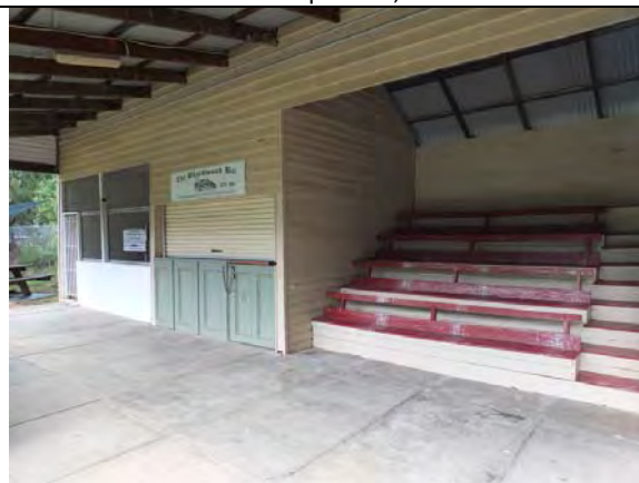
Photo 5: Detail of the east elevation of the timber pavilion, 2014.
