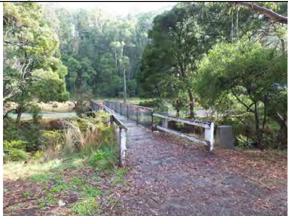
Photo 11: W.A. Matheson Bridge, looking north, 2014.
