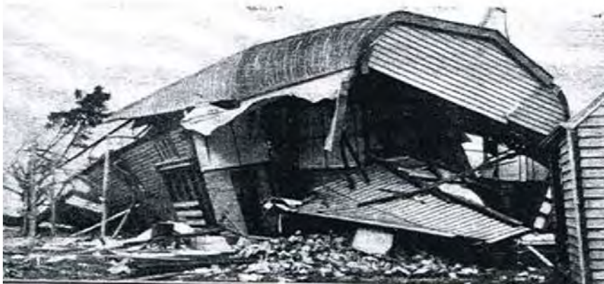
Figure 1: Rear wing of Mechanics' Institute destroyed by the cyclone in 1927.
