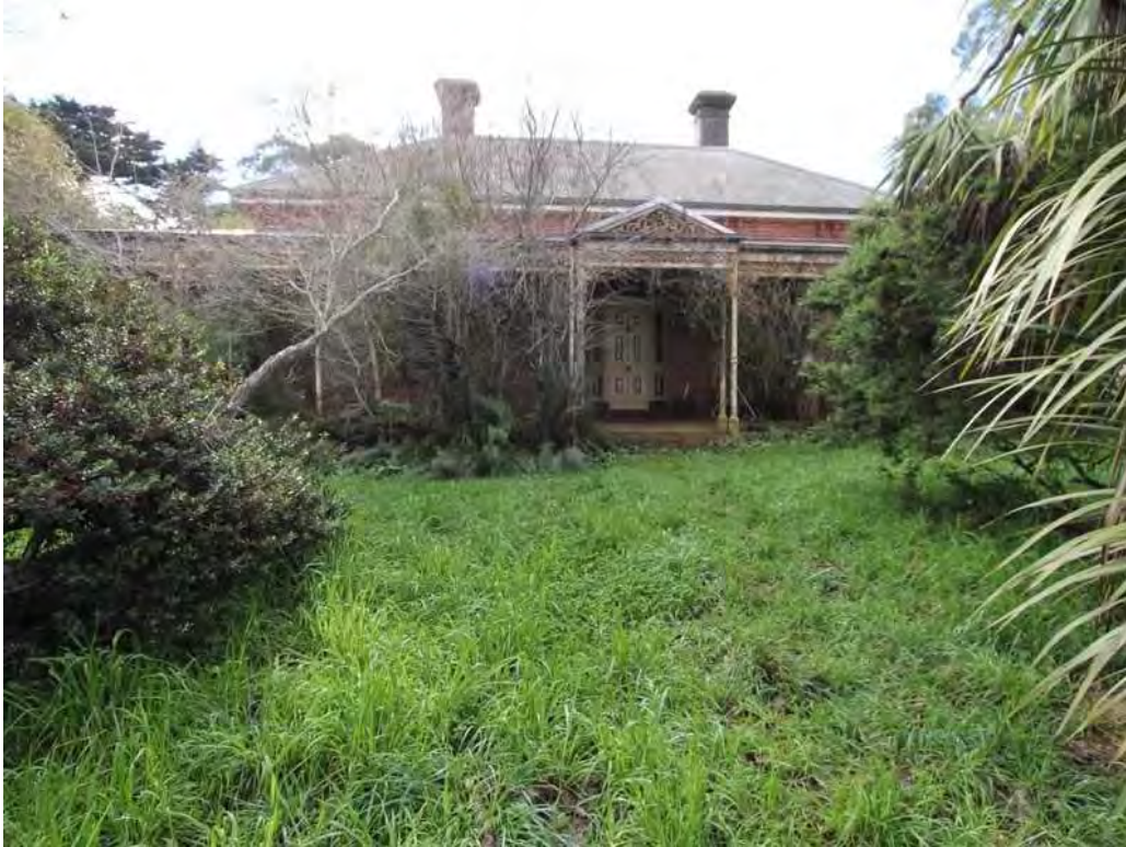
Photo 6: Front (south) elevation of main dwelling, 2012.
