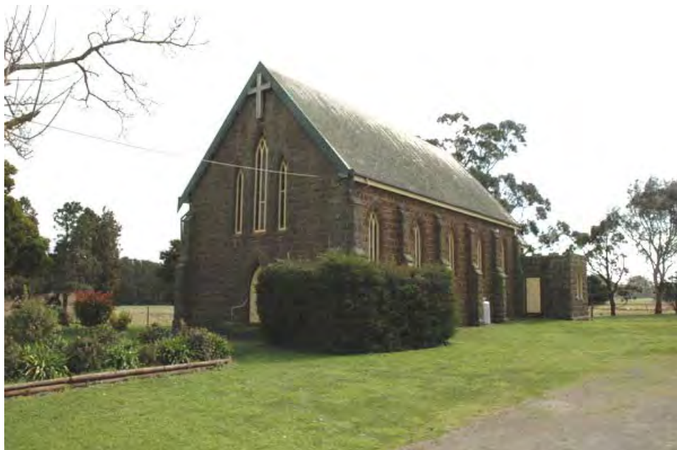
Photo 3: St. John's Anglican Church, front (south) and east elevations, showing projecting vestry addition at the rear, 2009.
