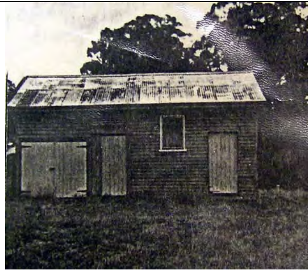
Figure 4: Former Police Stables & Forage Store, north elevation, January 1978.
