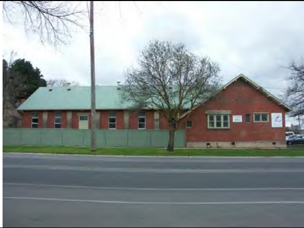
Former Ballarat North Progress Association Hall.
