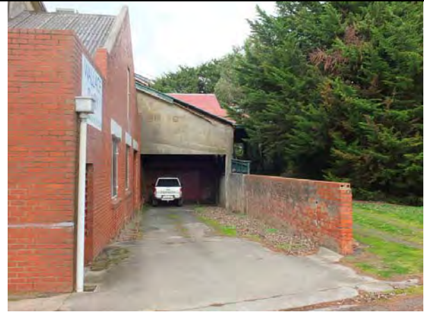
Photo 3: Former Butter Factory (Building 1), north elevation (west end), 2014. The projecting gable end represents the addition of 1922. The roof projecting above is the gambrel-roofed porte-cochere of 1908.
