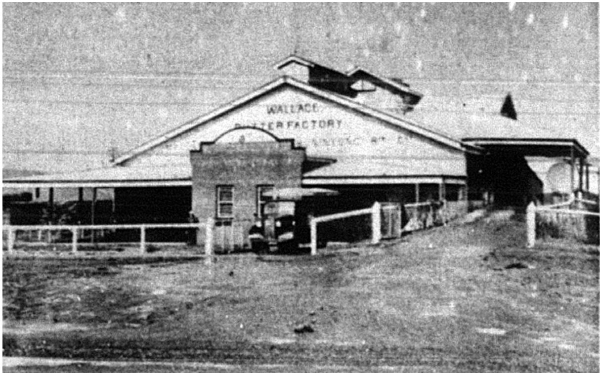
Figure 7: Butter factory, front elevation, showing two storey gabled attic addition behind the monitor light of the front gabled wing), 1939. Source: The Argus , 29 September 1939, p.18.
