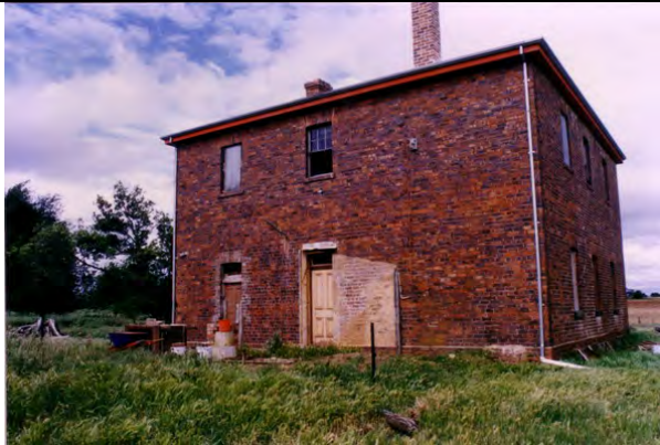
Figure 4: Oakvale', rear (west) elevation, 1998.
