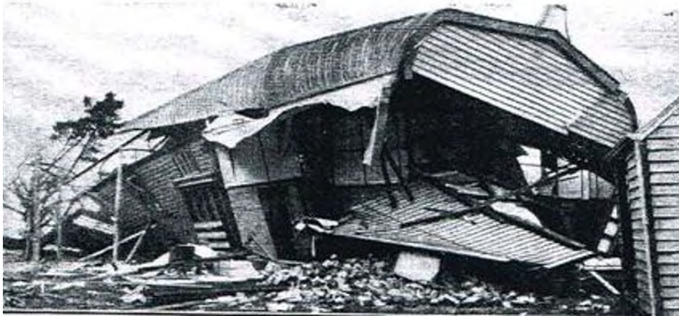
Figure 3: Mechanics' Institute, Bungaree Wallace Road, 1927, substantially damaged by a cyclone. Source: Bungaree History Walk at http://www.bungareehistorywalk.com/a-cyclone-destroys-the-hall.html .
