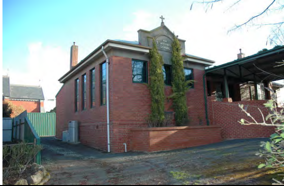
Photo 7: Former St. Michael's School, north elevation, 2009.
