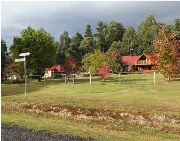
Photo 1: 'Beckett' property, showing the former police quarters & court house on the left, 2014.
