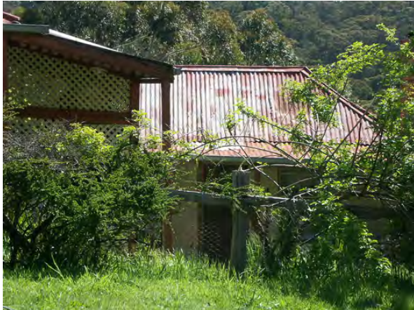
Photo 1: Front elevation of early dwelling on the side portion of the site, 2009.
