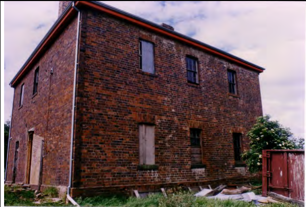
Figure 5: Oakvale', side (south) elevation, 1998.
