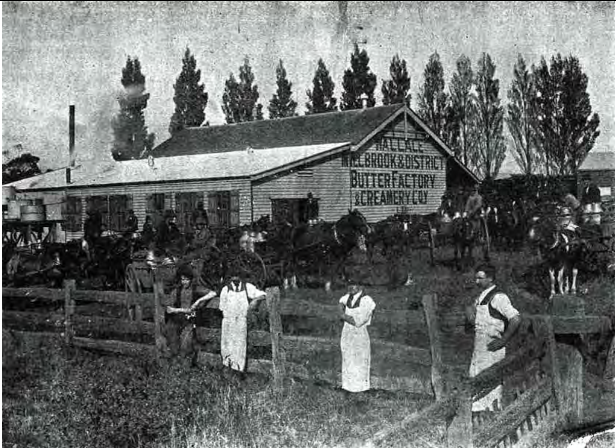
Figure 1: Original gabled and skillion building, Wallace Millbrook & District Butter Factory & Creamery, 1901.
