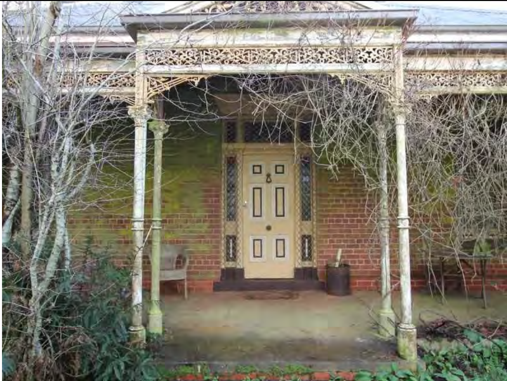
Photo 7: Detail of gabled verandah portico and main doorway behind, 2012.
