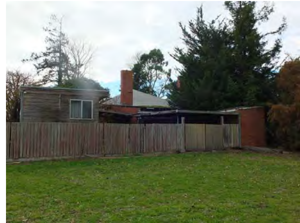
Photo 10: Brick Interwar Bungalow (Building 3), south elevation with rear early brick skillion outbuilding (right) and introduced timber outbuilding (left), 2014.
