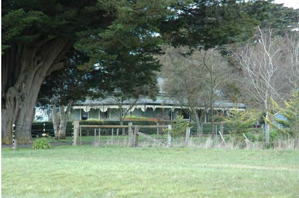
Photo 2: Dwelling, 634 Bungaree Wallace Road, front and side (west) elevations, 2009.
