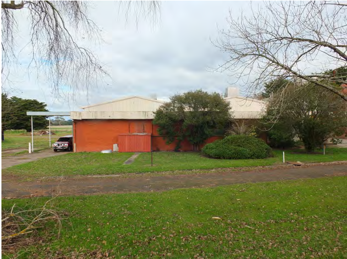
Photo 8: Former Cheese Factory (Building 2), north elevation, 2014.
