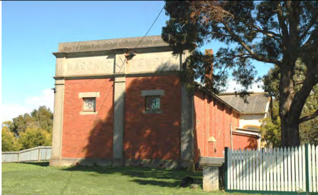
Photo 3: Masonic Temple, front (east) and side (north) elevations, 2009, with original “Masonic Temple” lettering and masonic square and compass symbol on the parapet.
