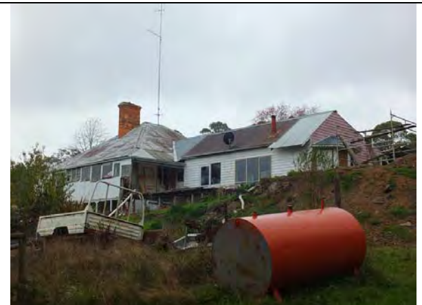
Photo 4: Dwelling from Warner Street (west and south elevations), 2014.
