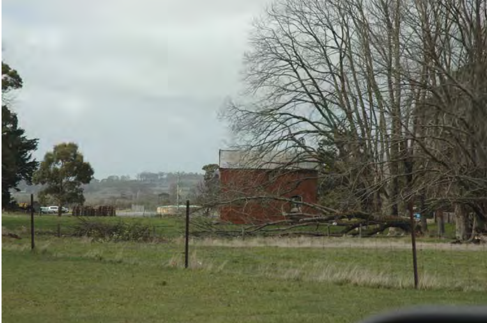
Photo 2: Former stables, 4 Erin Court, west elevation, 2009.
