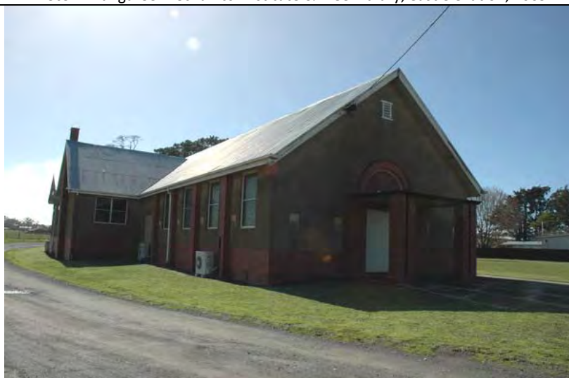
Photo 3: Bungaree Mechanics' Institute & Free Library, south & west elevations, 2009.
