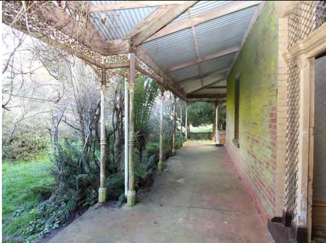
Photo 8: View under front verandah (looking west), 2012.
