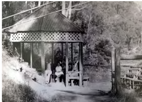
Figure 9: North pavilion, c.1937. Source: Blackwood & District Historical Society.
