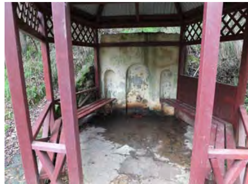
Photo 2: North Pavilion, 2014, showing the rendered masonry wall with water outlet.
