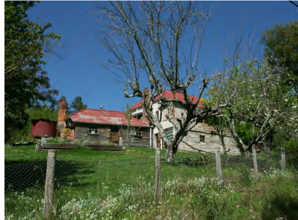
Photo 3: Rear elevations of early and later dwellings, 2009.
