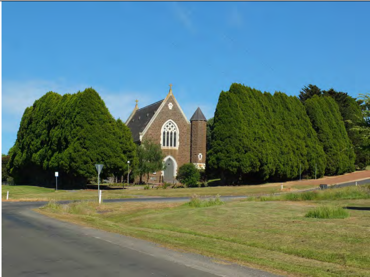
Photo 3: St. Patrick's Catholic Church, showing perimeter trees from the south-east corner, 2014.
