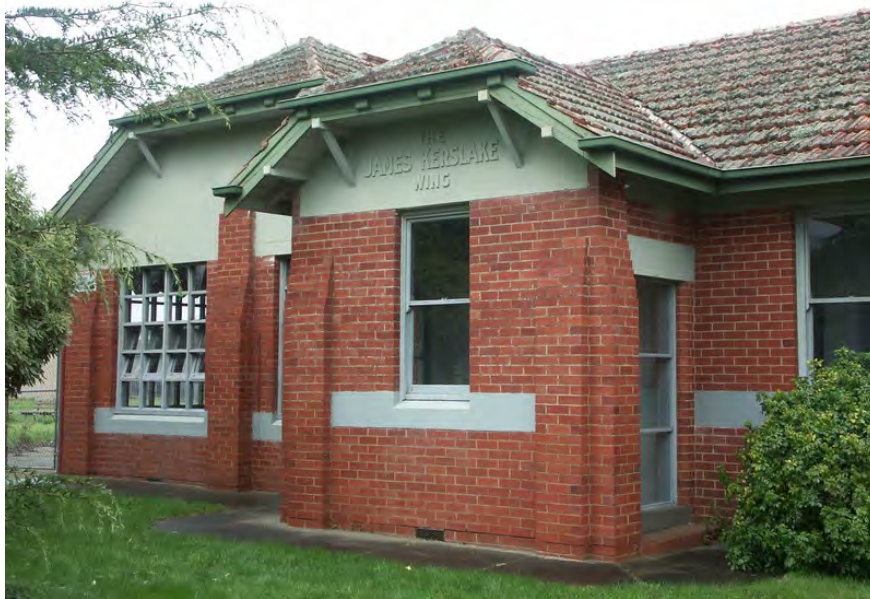
Figure 2: James Kerslake Wing (built 1939) of the former Toddlers' Block, Ballarat Orphanage, Ballarat East, showing similar, contextually unusual projecting wings with jerkin head roof forms with terra cotta tile roof cladding and face brick wall construction and roughcast render in the gable ends. Source: David Rowe, 2011.
