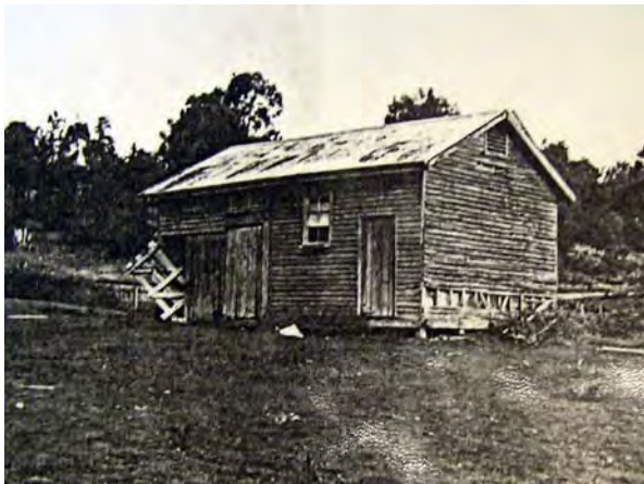
Figure 3: Former Police Stables & Forage Store, north and west elevations, November 1975.
