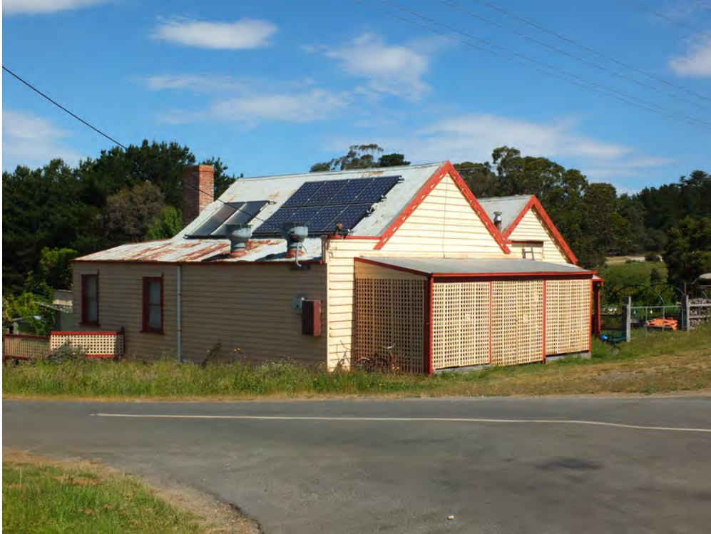
Photo 2: Dwelling and former Store, north and west elevations, 2014.
