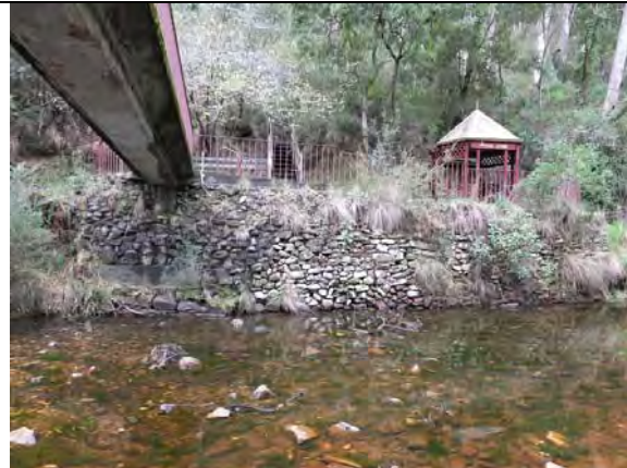
Photo 6: Random stone retaining wall forming the north bank of the Lerderderg River, 2014.
