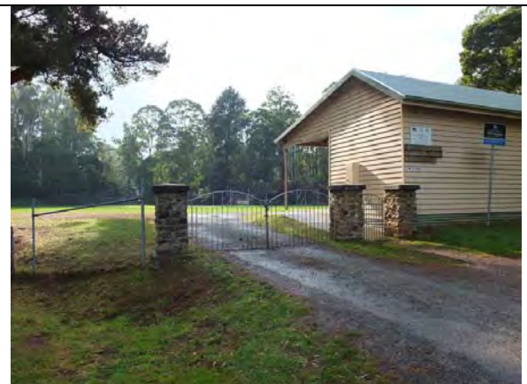
Photo 6: Random rubble gate piers and metal gates, 2014.
