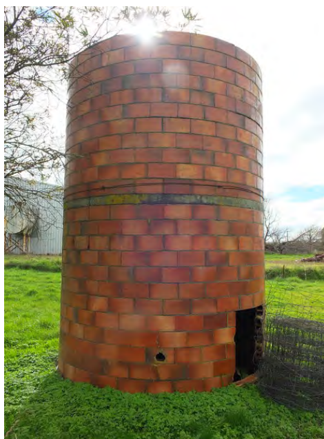
Photo 14: Terra cotta tank, south and east elevations, 2014.
