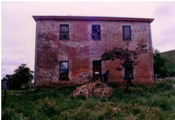
Figure 2: 'Oakvale', front (east) elevation, 1998.
