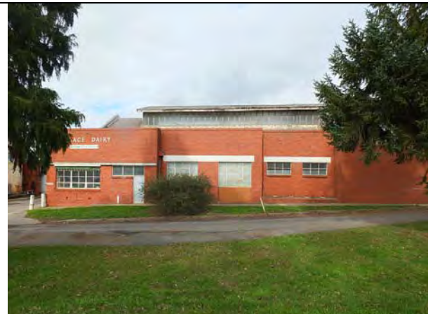
Photo 7: Former Butter Factory (Building 1), 2014. North elevation of the parapeted wing of the additions of the 1940s-50s.
