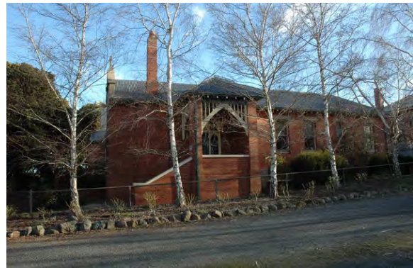
Photo 6: Former St. Michael's Presbytery, north elevation, 2009.
