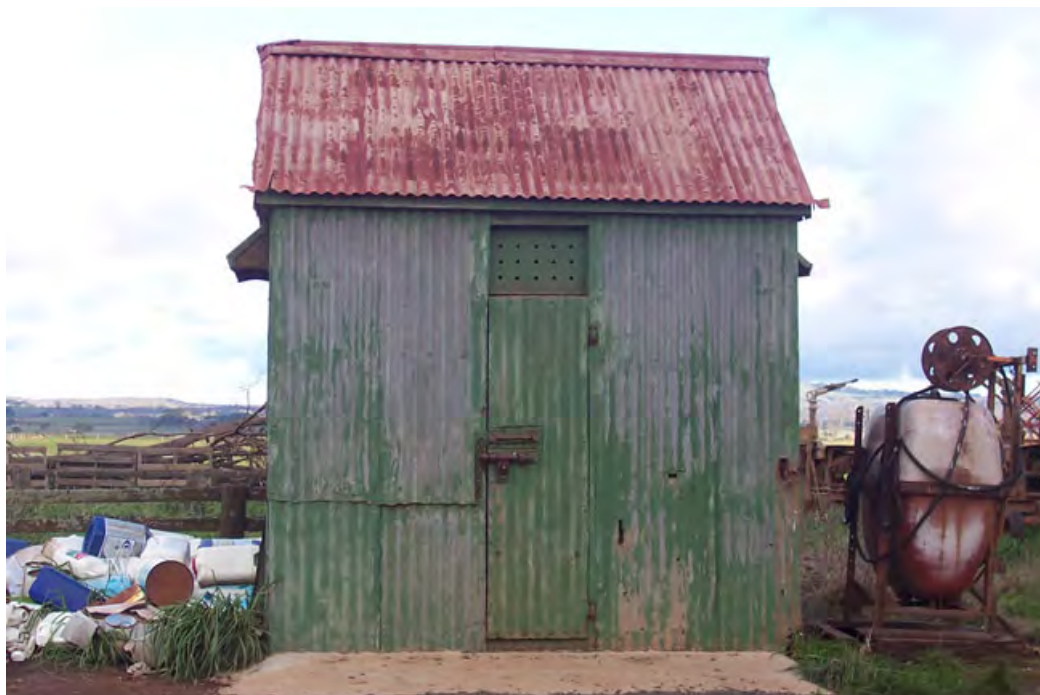
Figure 7: Former Warrenheip Lock Up, Dunnstown. Source: Dianne Cahir, Dunnstown, 2010.
