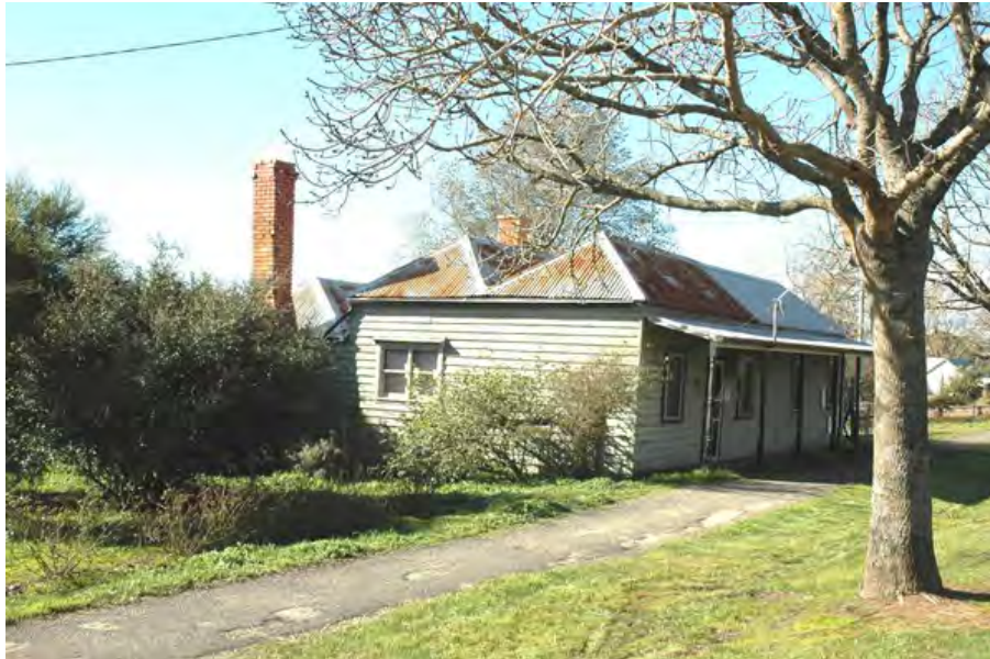
Photo 2: Dwelling and former store and bakery, west and south (front) elevations, 2009.
