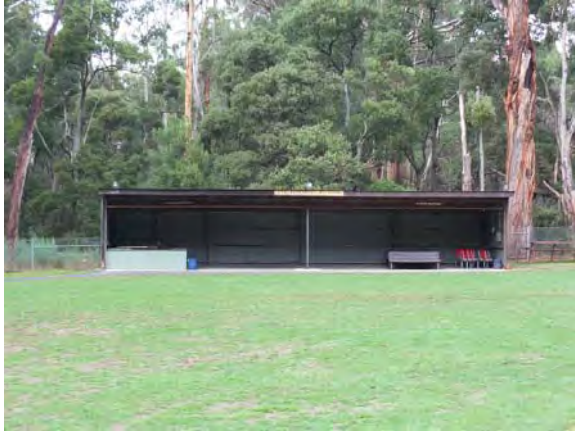
Photo 7: Les Armstrong Pavilion, located on the south side of the recreation ground, 2014.
