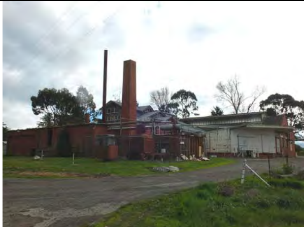
Photo 4: Former Butter Factory, south and east elevations, 2014. The elevated gabled wing behind the chimney stack is the addition of the 1930s, the lower portions (including the lower gabled form on the right side) being the original building of 1908.
