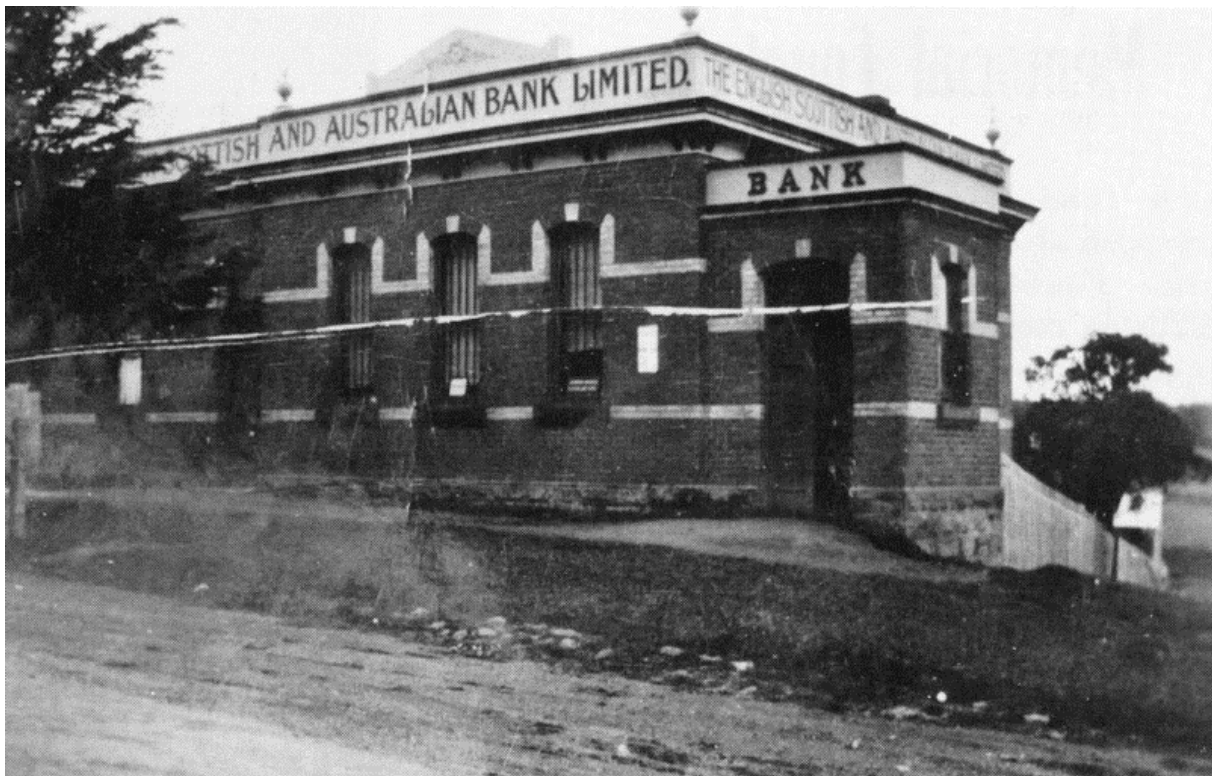
Figure 2: Former London Chartered Bank (when the ES & A Bank), n.d. [c.1930], 64 Main Street, Gordon.
