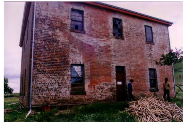
Figure 3: 'Oakvale', front (east) elevation, 1998.
