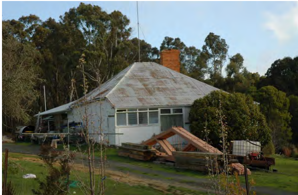
Photo 1: Dwelling from Terrill Street (north & east elevations), 2009.
