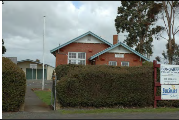
Figure 6: Bungaree Primary School, 2009, prior alterations & additions at front. Source: Wendy Jacobs.
