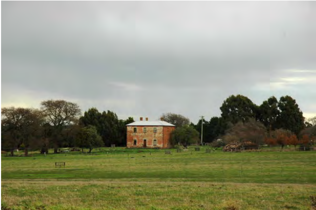
Photo 2: 'Oakvale' front (east) elevation, viewed from Boundary Road, 2009.
