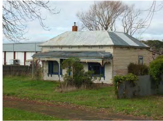
Photo 12: Late Victorian timber dwelling (Building 5), north and west elevations, 2014.
