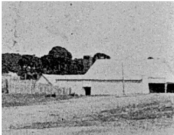
Figure 1: Distant view from corner of Main and Russell Streets of the dwelling store at 32 Russell Street, n.d. [pre 1913] Source: Museum Victoria online, image MM001850.
