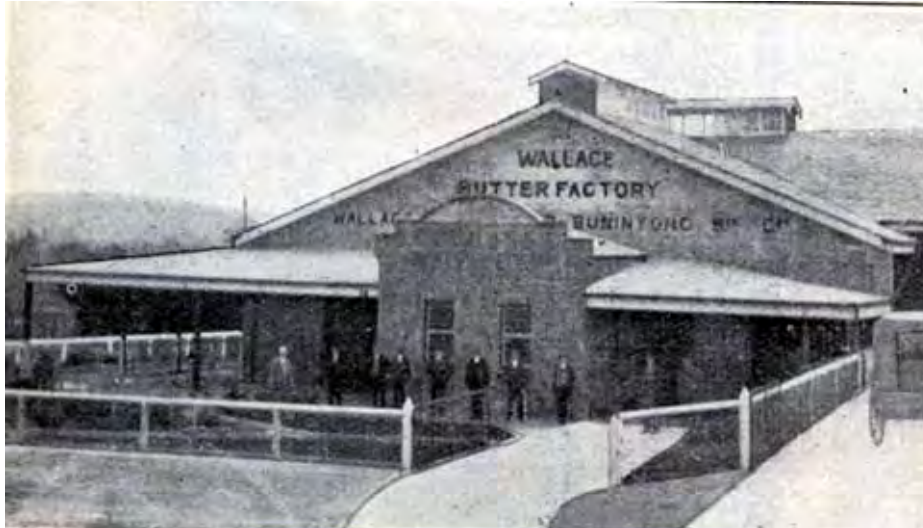
Figure 6: Butter factory, front elevation, showing the addition of the central parapeted bay at the front, c.1928.
