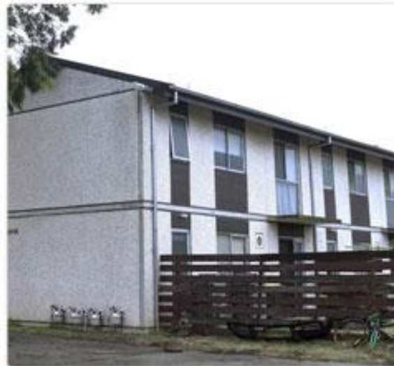
The original Young Street housing
