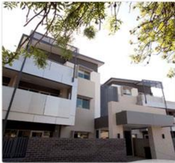
New public housing at Young Street
