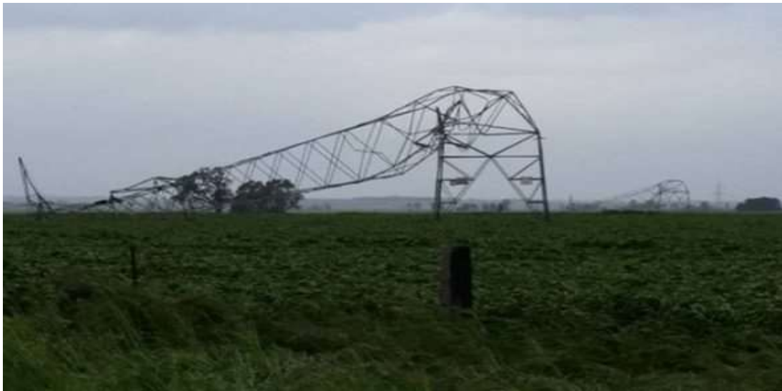
Figure 16: Fallen 275 kV tower in South Australia 14
