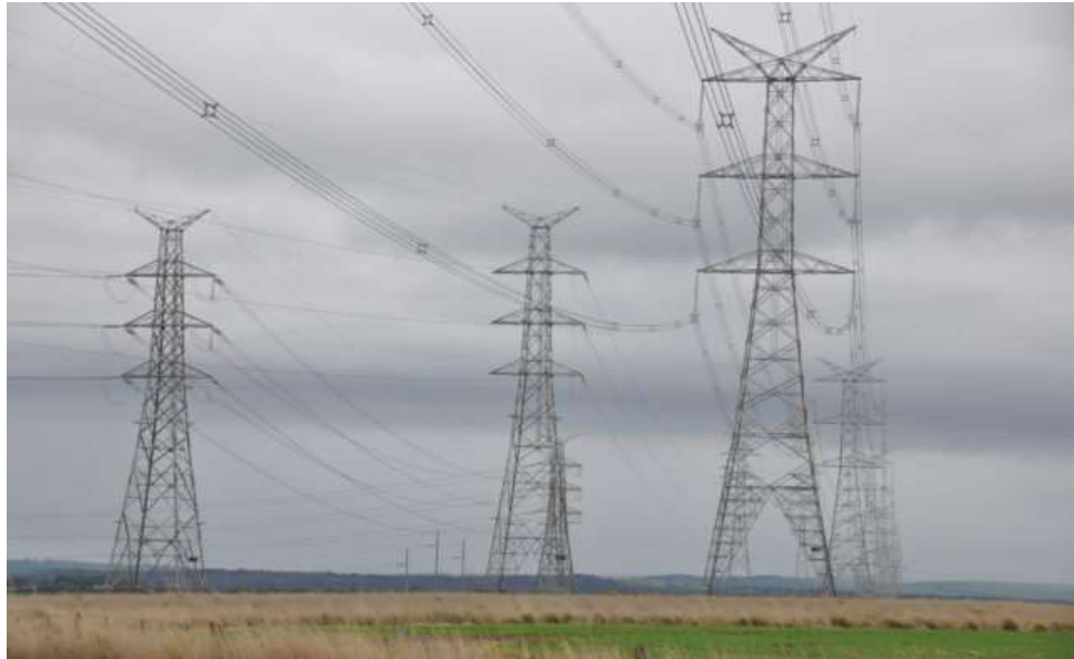
Figure 5: 500 kV double circuit overhead lines and towers (series on the right) 8
