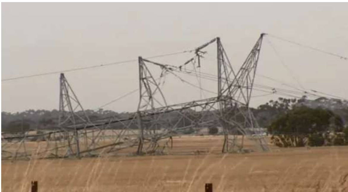
Figure 13: Fallen 500 kV double circuit tower (Moorabool to Haunted Gully and Mortlake) 11
