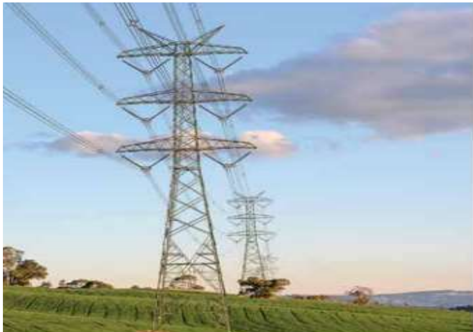
Figure 6: 500 kV double circuit overhead lines and towers [3]
