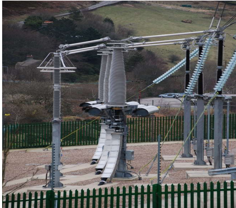
Figure 10: 400 kV underground cable outdoor termination at a transition station
