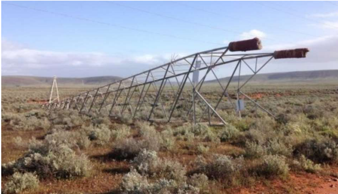
Figure 17: Fallen 275 kV tower in South Australia 15
