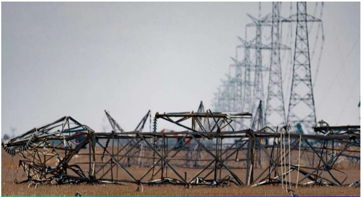
Figure 12: Fallen 500 kV double circuit tower (Moorabool to Haunted Gully and Mortlake) 10
