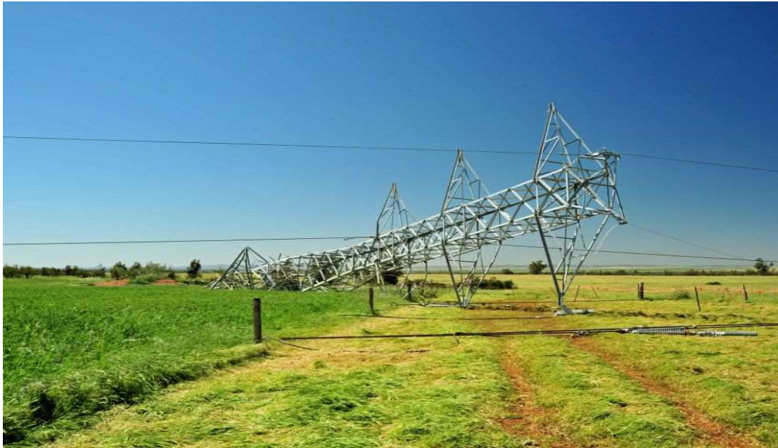
Figure 15: Fallen 275 kV tower in South Australia 13
