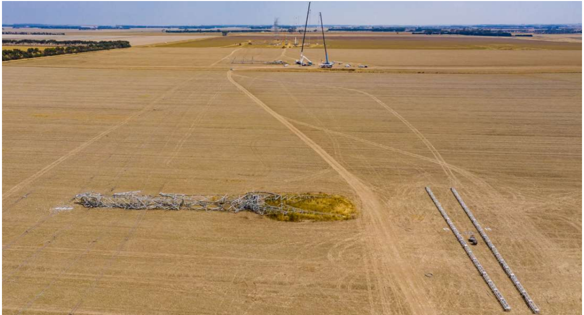
Figure 14: Fallen 500 kV double circuit tower (Moorabool to Haunted Gully and Mortlake) 12
