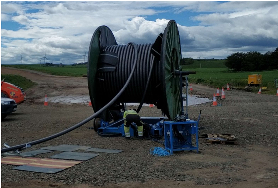
Figure 38: Cable being pulled from a drum that is mounted on a motorised stand
