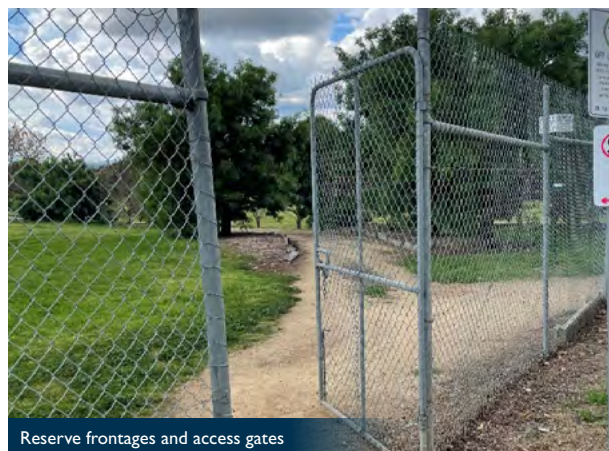
Reserve frontages and access gates
