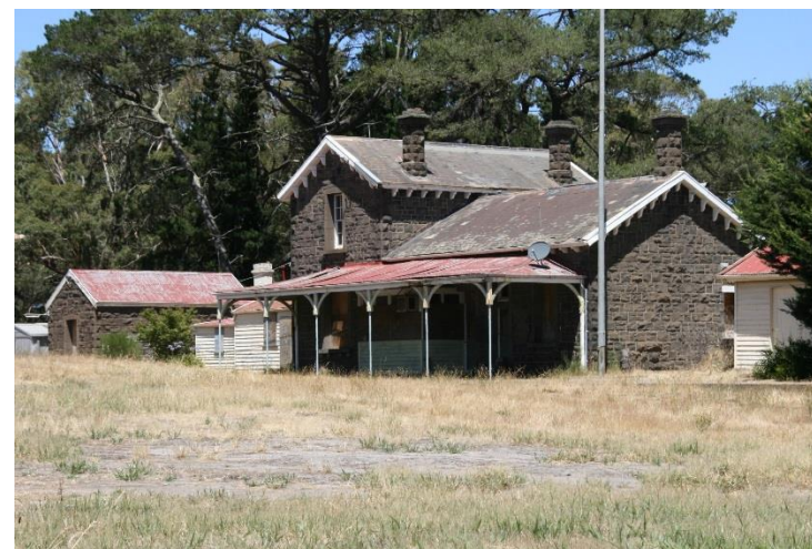
Photo 1 Former Train Station building at Lal Lal
