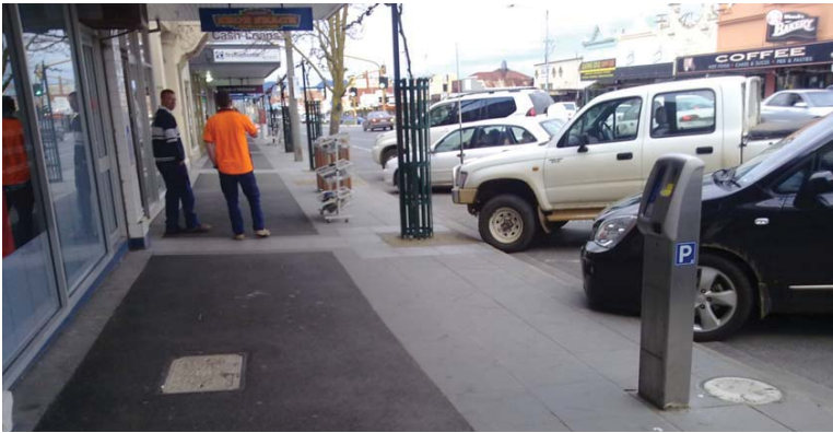
Bluestone at back of kerb, with asphalt along building line
