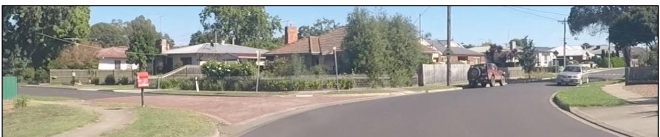
Figure 4-5 Existing Threshold Treatment on Dugdale Street in Bacchus Marsh
