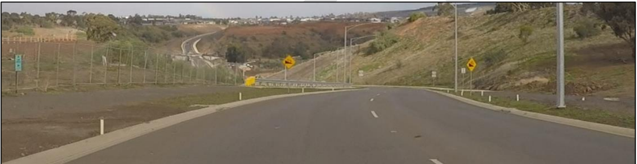
Figure 4-3 Halletts Way facing south
