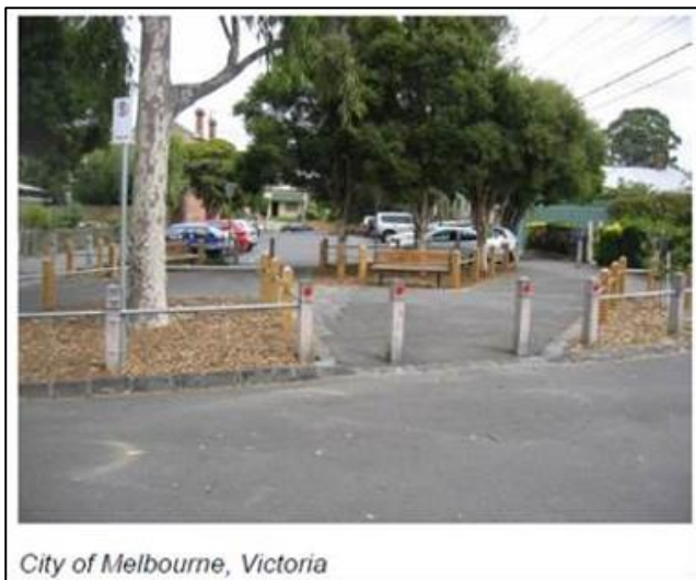
Figure 3-7 Full Road Closure
