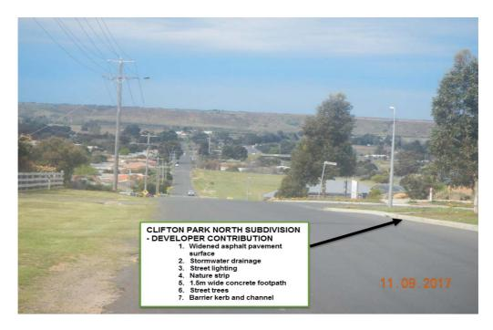
Works for stage 3, on the southern side of Holts Lane abutting the development west of Meridie Way to Halletts Way will be constructed similar to the existing developments in Stage 1 & 2. The time frame for development of this stage is unknown as no development proposal has been submitted to Council.
