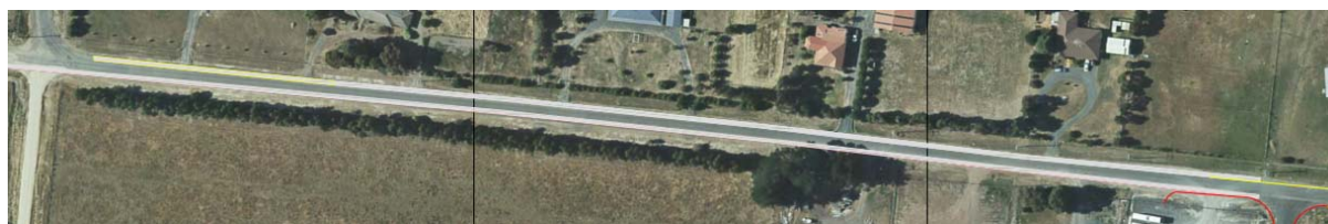
Gillespies Lane, Ballan – shoulder sealing
