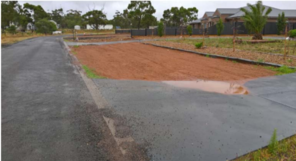
Figure 2: filled swale drain in front of a property in Carberry Drive, Hopetoun Park.
