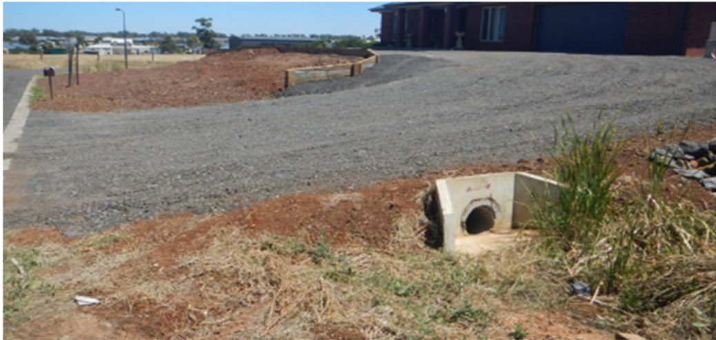
Figure 8: filled swale drain in front of a property at Eden Crescent, Hopetoun Park.
