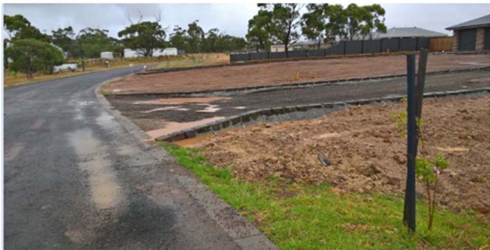
Figure 3: filled swale drain in front of a property in Carberry Drive, Hopetoun Park
