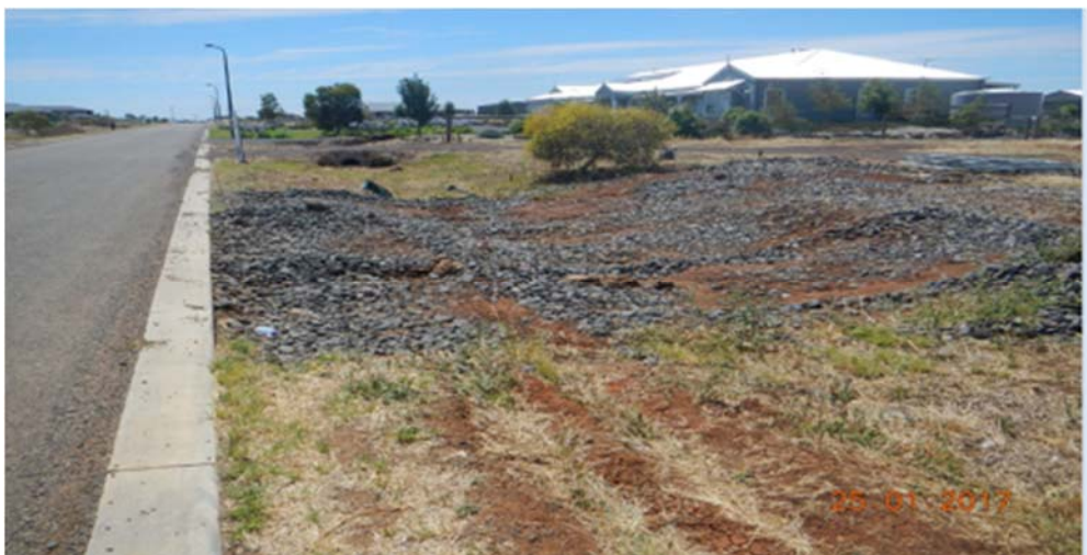
Figure 9: additional crossover constructed with no endwalls and without a permit from Council. Swale drain backfilled in front of a property in View Gully Road, Hopetoun Park.
