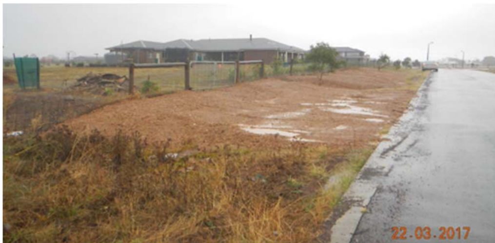
Figure 9: additional crossover constructed with no endwalls and without a permit from Council. Swale drain backfilled in front of a property in View Gully Road, Hopetoun Park.
