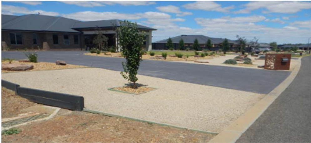
Figure 5: filled swale drain, construction of brick letterbox over nature strip and landscaping in front of a property in Mia Bella Drive, Hopetoun Park.
