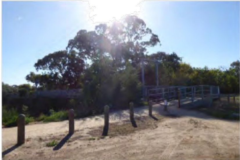
G - Pedestrian bridge crossing the Werribee River at the northwest corner of the development plan area
