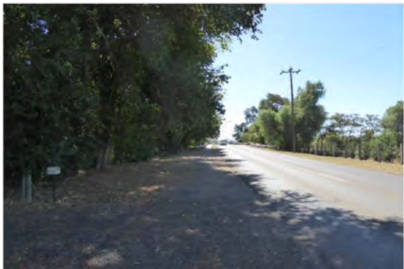
R - Fiskin Street Bridge crossing the Werribee River to the northeast of the development plan area
