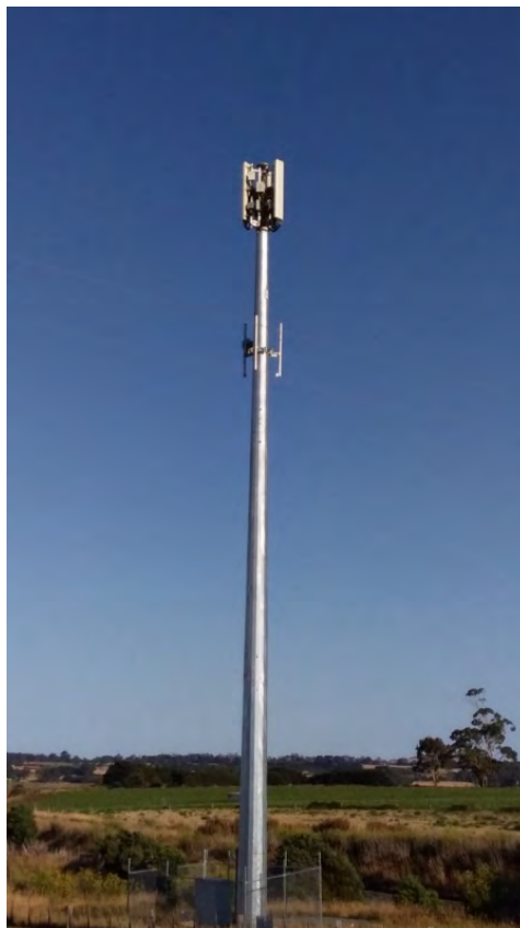
Photo: The telecommunication tower off Sullivans Road in Millbrook, Victoria.
