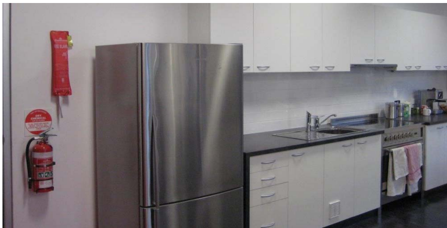
Figure 4: Installation of Fire Extinguisher and Fire Blanket in Kitchen
