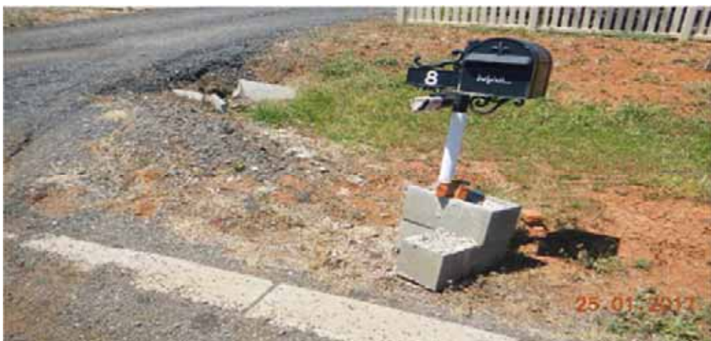
Figure 6: damaged end wall, concrete filled blocks around letterbox and backfilled swale drain in front of a property at View Gully Road, Hopetoun Park.
