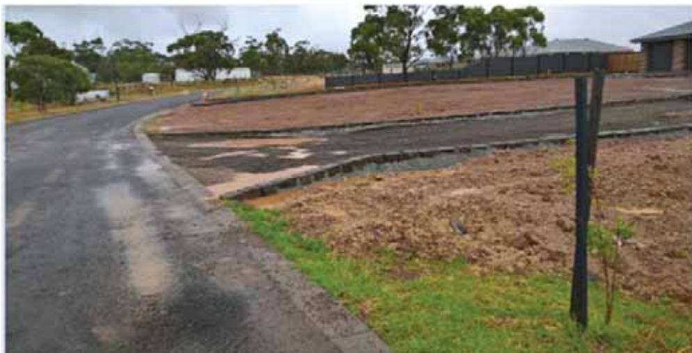
Figure 3: filled swale drain in front of a property in Carberry Drive, Hopetoun Park
