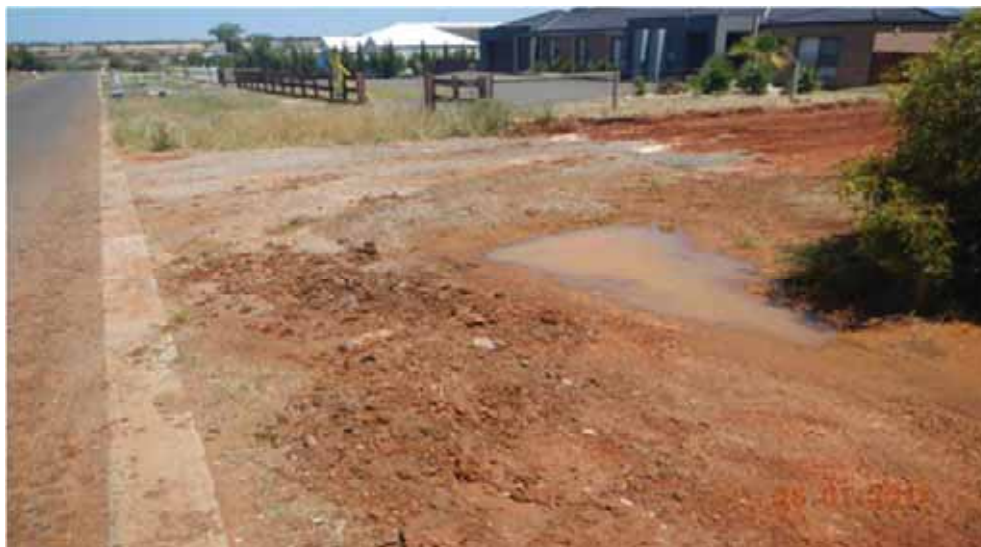
Figure 11: at Thomas Drive, Hopetoun Park, an additional crossover was built without stormwater pipes and endwalls. The swale drain has been filled with soil.
