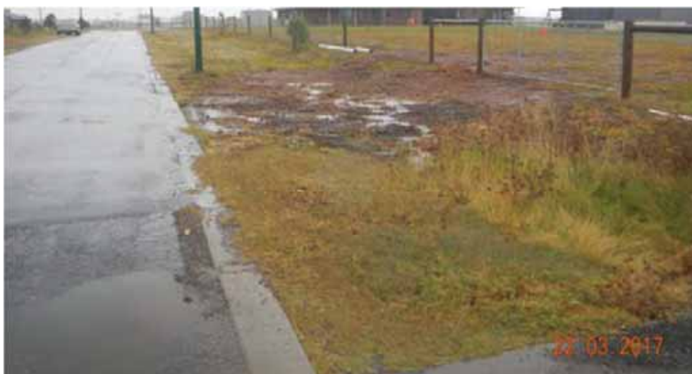
Figure 11: at Thomas Drive, Hopetoun Park, an additional crossover was built without stormwater pipes and endwalls. The swale drain has been filled with soil.
