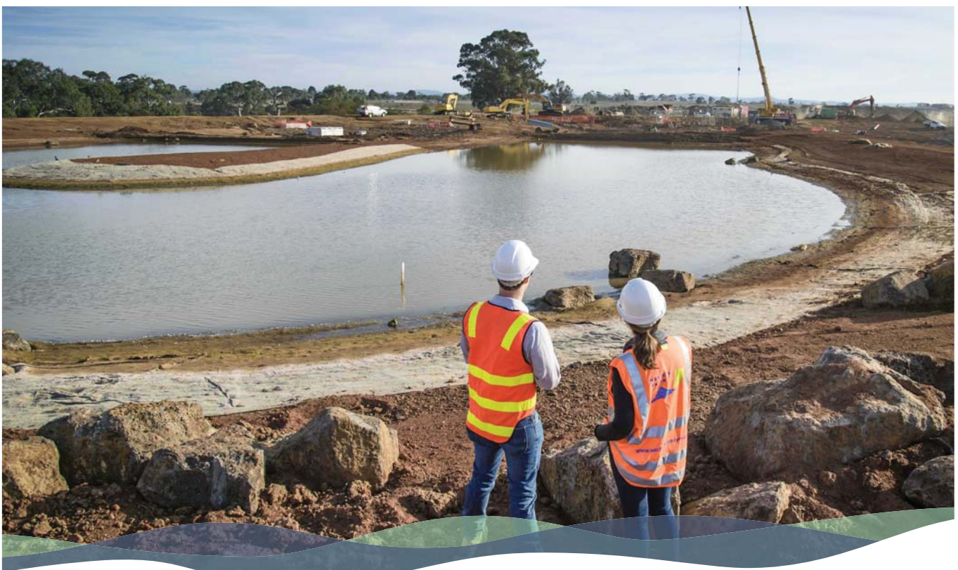
Toolern wetland. Courtesy: Western Water
