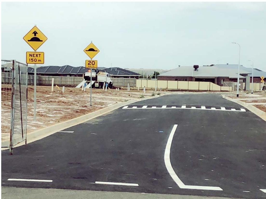
Near Burrbridge Drive Intersection
