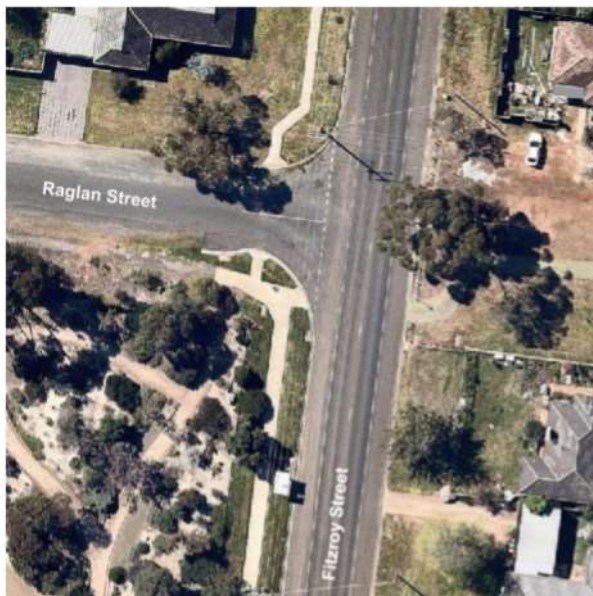
Figure 4-3 Fitzroy Street at the intersection with Raglan Street
