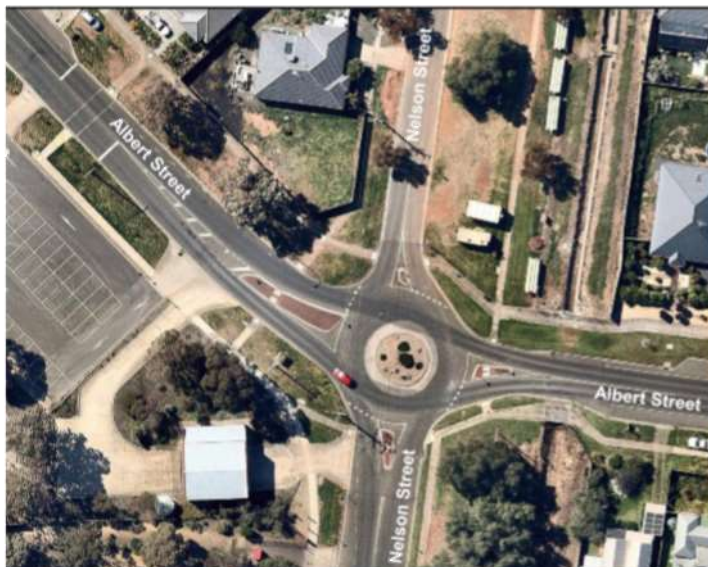
Figure 4-2 The roundabout at the intersection of Albert Street and Nelson Street
