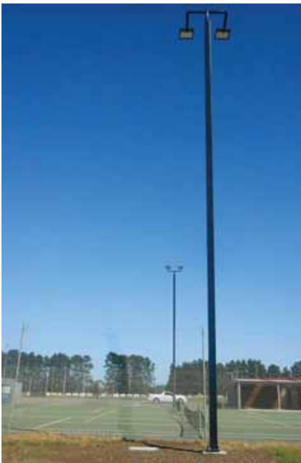
Dunnstown Recreation Reserve lighting
