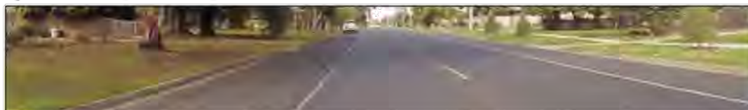
Figure 4-6 Fitzroy Street, Looking south
