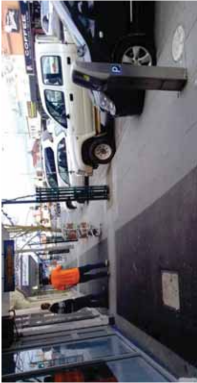
Bluestone at back of kerb, with asphalt along building line
