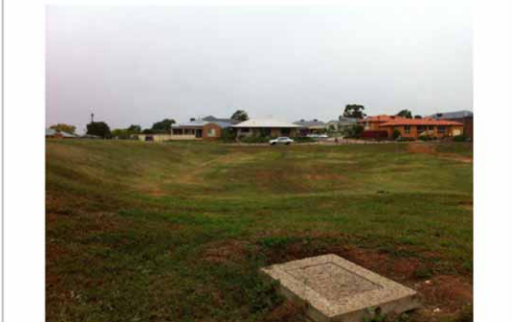
Photo 14: Retarding Basin on Masons Lane Drain
