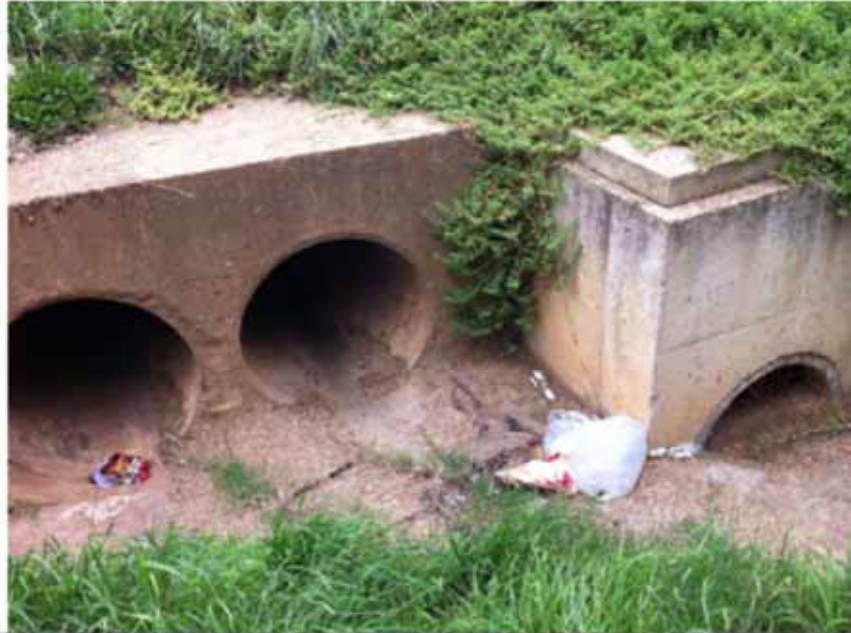
Photo 1: Holts Lane Culvert near Halletts Way
