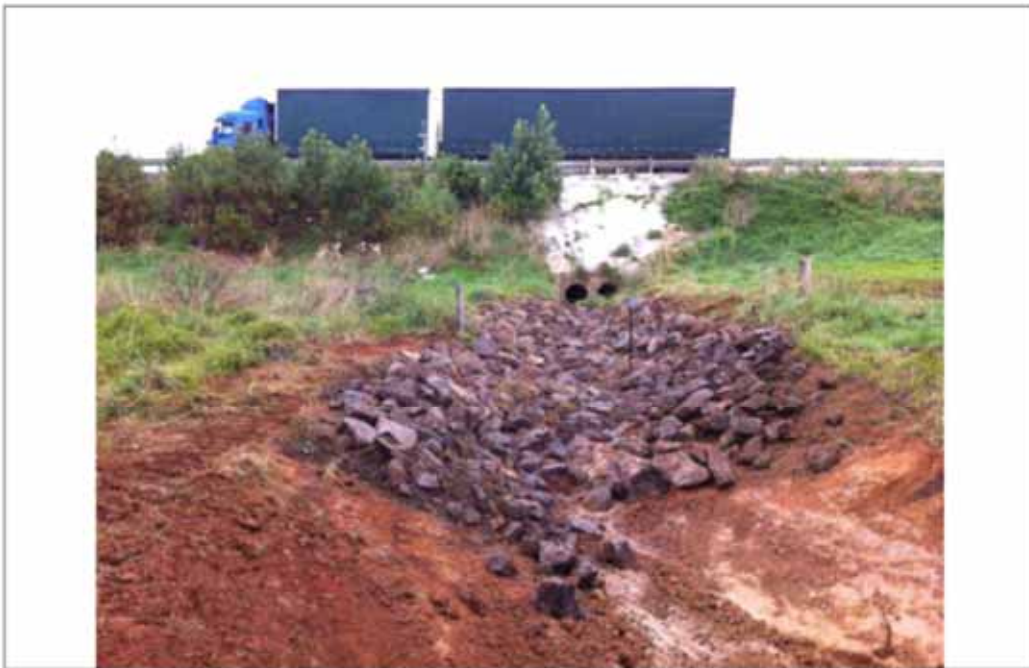
Photo 21: Masons Lane Waterway looking upstream from south of Western Freeway
