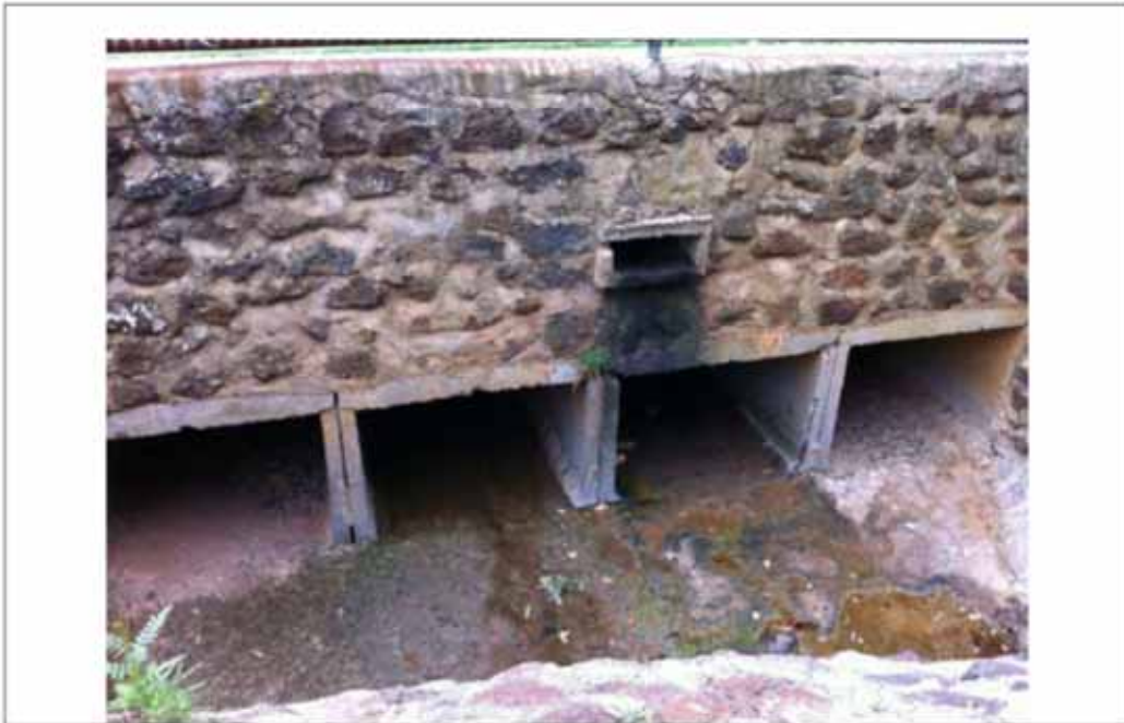
Photo 17: Culverts Downstream of Retarding Basin on Masons Lane Drain
