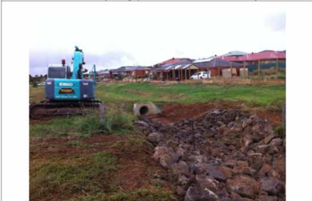
Photo 22: Masons Lane Waterway looking downstream from south of Western Freeway
