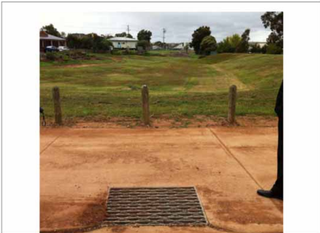
Photo 15: Retarding Basin on Masons Lane Drain
