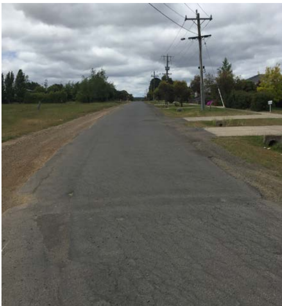
Sealed section (southern end), facing north
