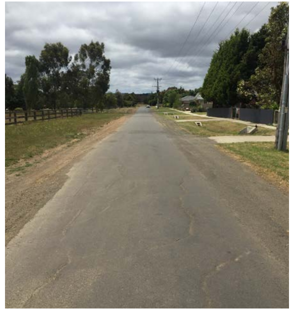
Sealed section (midway), facing north
