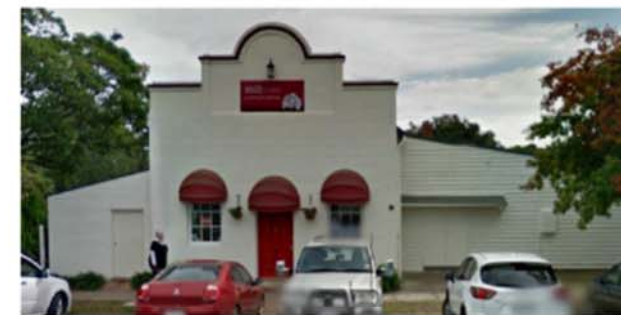
PROPERTY TO THE NORTH, ACROSS THE ROAD, AT 94 INGLIS STREET WHERE MILL ROSE GUITING AND GALLERY IS SITUATED
