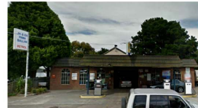
ADJOINING PROPERTY TO THE EAST AT 95 INGLIS STREET WHICH CURRENTLY HOLDS PAMA MOTORS BALLAN
