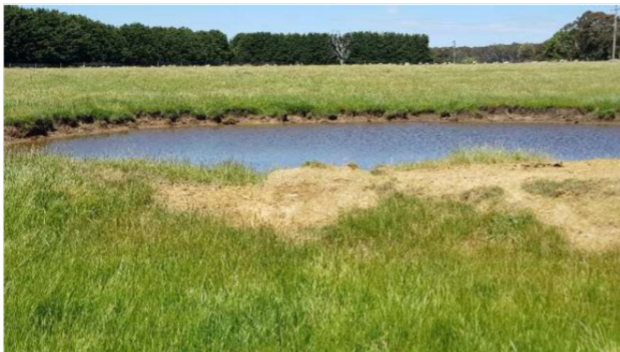
Figure 8: Dam at 139 Pound Creek Road, Navigators
