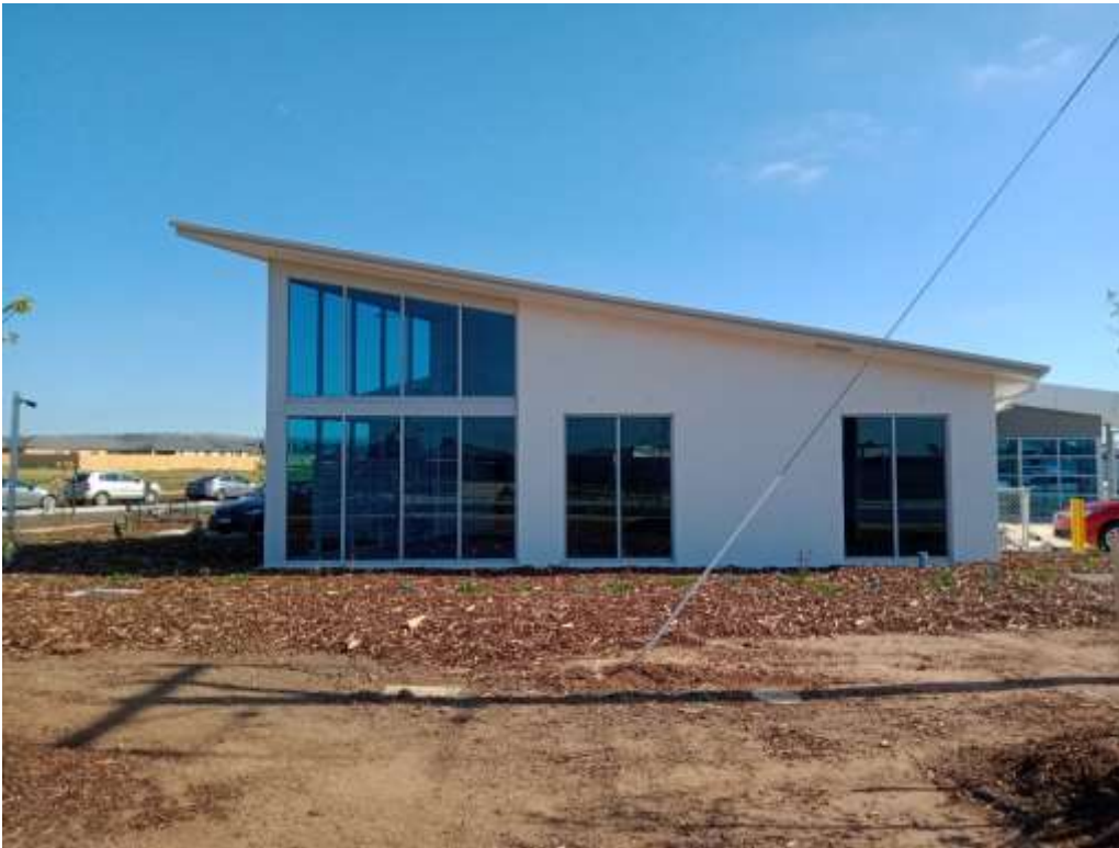
View of the dispensary area. Taken 22 October 2019.
