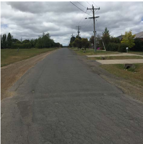
Sealed section (southern end), facing north
