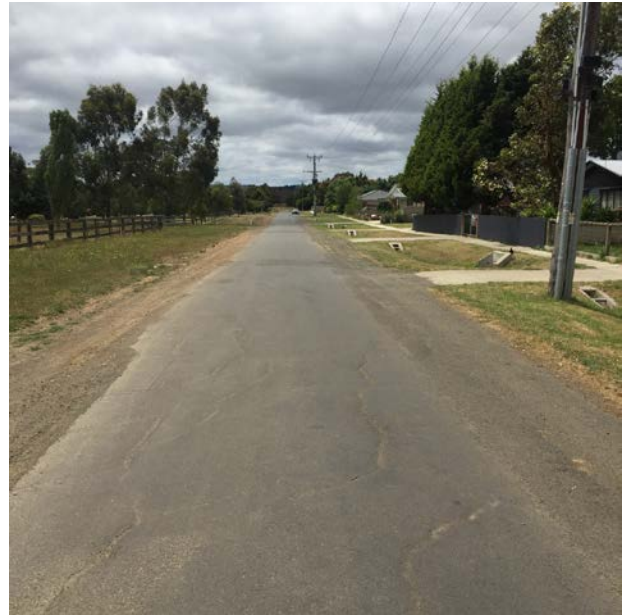
Sealed section (midway), facing north
