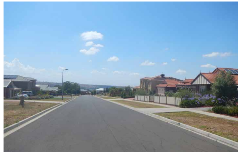
Non existent street plantings with a one sided footpath.
