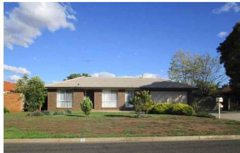
Brick dwelling with moderate landscaping and generous front setback.
