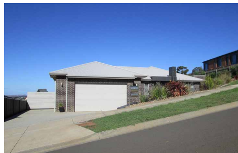
Site cuts and retaining walls feature throughout the precinct.
