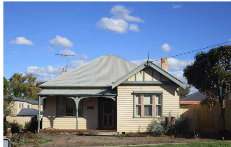
Weatherboard dwellings with traditional front setbacks dominate the precinct.
