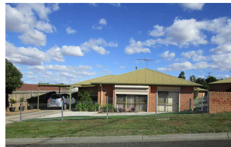
Conventional dwelling with minimal landscaping and metal fencing which is present throughout this precinct.
