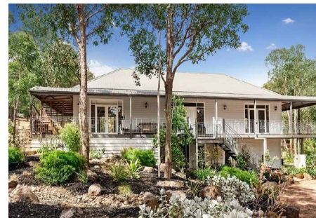
Dwelling sympathetic to the site topography and avoiding significant site cut.
