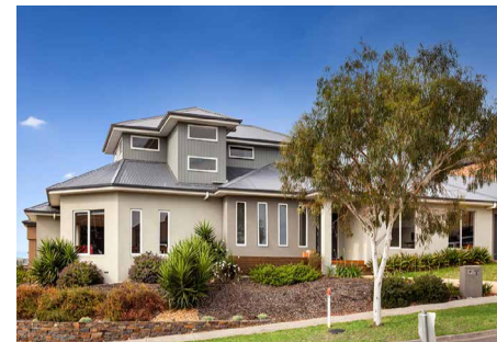
Articulated two storey dwelling on a corner allotment that has a strong presence to both streets.
