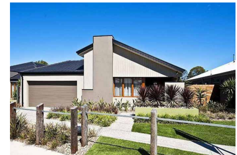
Contemporary dwelling with skillion roof that complements many roof forms within the precinct.
