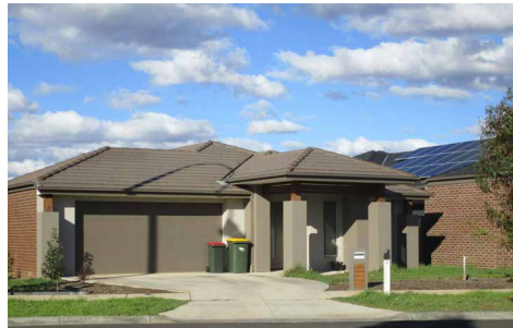
Contemporary dwelling with landscaping still establishing and a conventional front setback.
