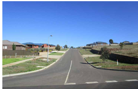
Streetscape deficient of landscaping.
