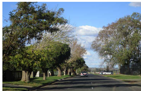
Wide road reserve, with established street tree plantings and a single sided footpath network.
