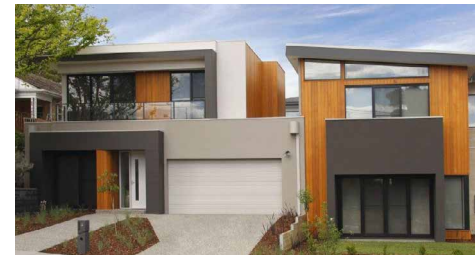
Multi-dwelling development on a corner lot, with vehicular access from both streets.
