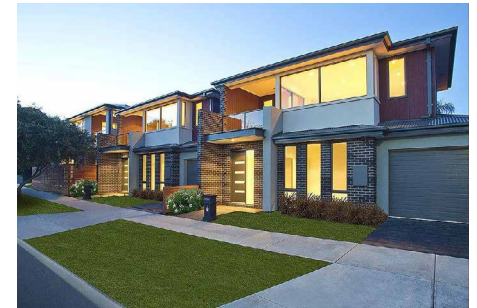
Contemporary multi-dwelling development that uses a mix of building materials. (Increased Residential Growth Areas).
