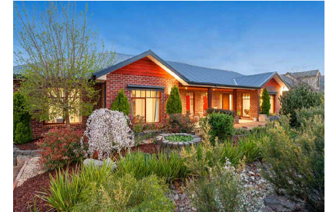
Modest dwelling set behind landscaped gardens.
