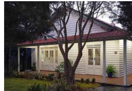
Dwelling with a generous front setback which has landscaping and built form materials that compliment the precinct.
