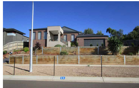
Contemporary dwelling with significant retaining walls and site cuts.
