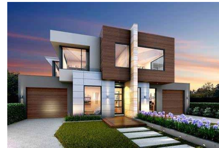
Well articulated contemporary multi-dwelling development.
