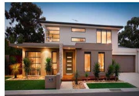
Articulated double storey dwelling.
