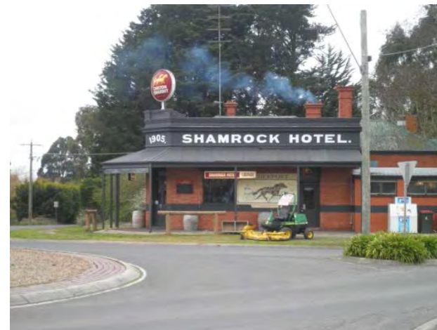
Shamrock Hotel, Old Melbourne Road, Dunnstown
