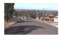
**PAVEMENT:** Structural portion of road, made up of compacted crushed rock or gravel.
