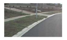
**BARRIER KERBS:** Straight, upright concrete edge that separates the road from the road side or footpath. Not driveable.
