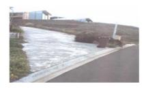
**SEMI MOUNTABLE KERBS:** Rolled concrete edge that separates the road from the roadside or footpath. Semi driveable.
