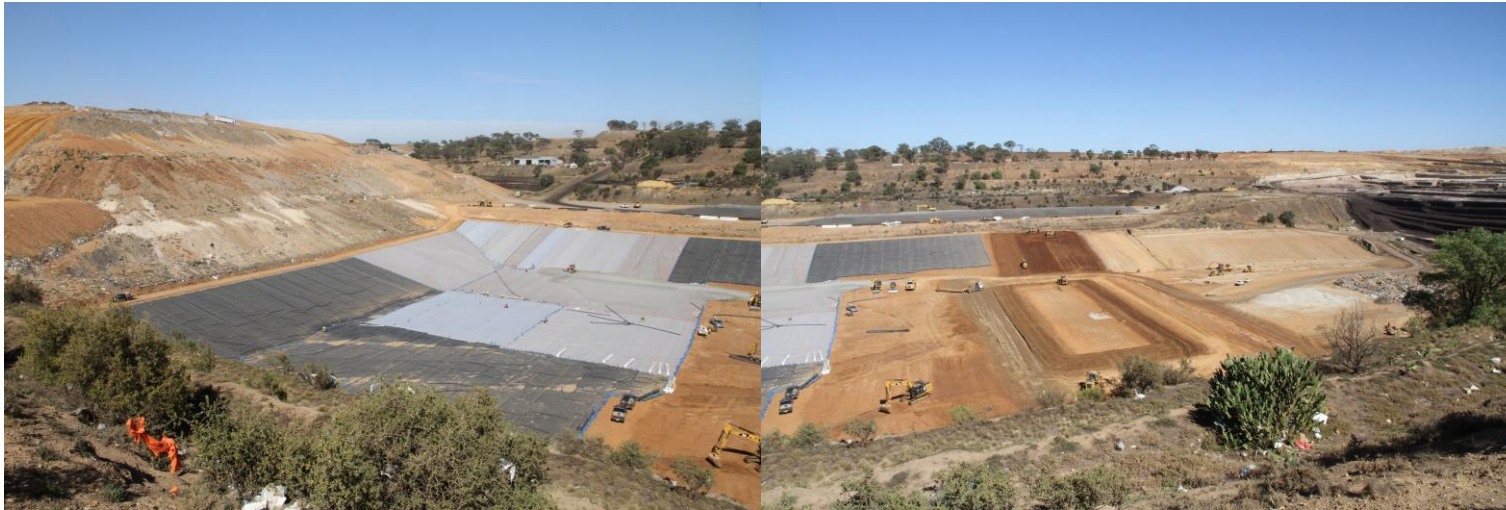
Photograph 5 Maddingley WRR Hub from the eastern edge on Cummings Road showing the completed Stage 1 (left photograph) and Stage 2 landfill cell construction (right photograph), January, 2019.
