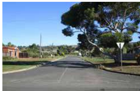
Wide road reserve, with no footpaths.
