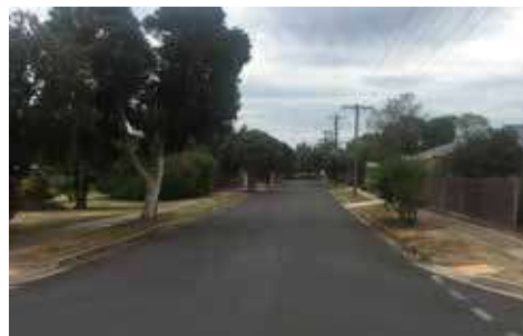
Wide road reserve, with inconsistent street tree plantings and a two sided footpath network.
