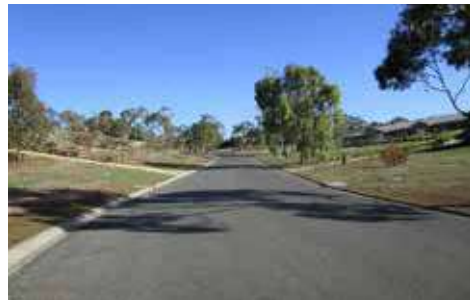
A curvilinear street network with no footpaths and wide road reserves.
