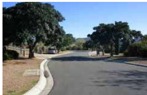
Wide road reserves with inconsistent street trees that are still maturing.
