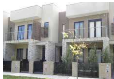
Multi-dwelling development that is well articulated and uses a mix of building materials.
