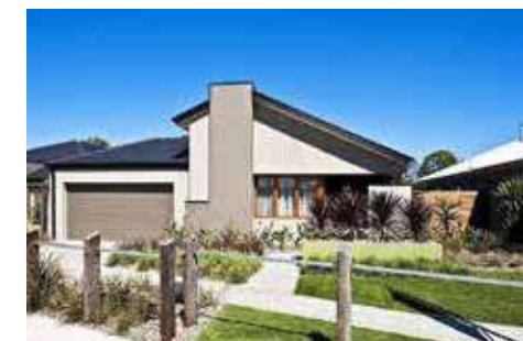
Contemporary dwelling with skillion roof that complements many roof forms within the precinct.
