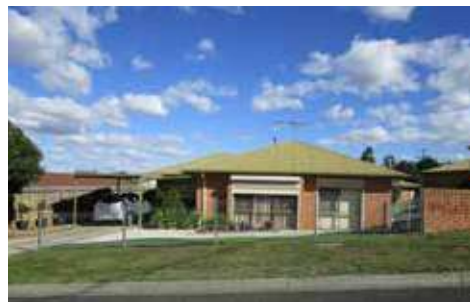
Conventional dwelling with minimal landscaping and metal fencing which is present throughout this precinct.
