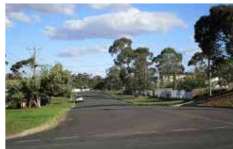
Wide road reserve, with inconsistent street tree plantings and no footpath network.
