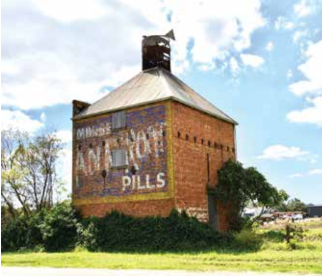
Chicory Kiln before the restoration, note the overgrown vegetation, weathered timber and top vent.
