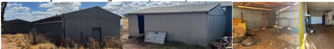
Former Pony Club & storage sheds (BMRRR)
