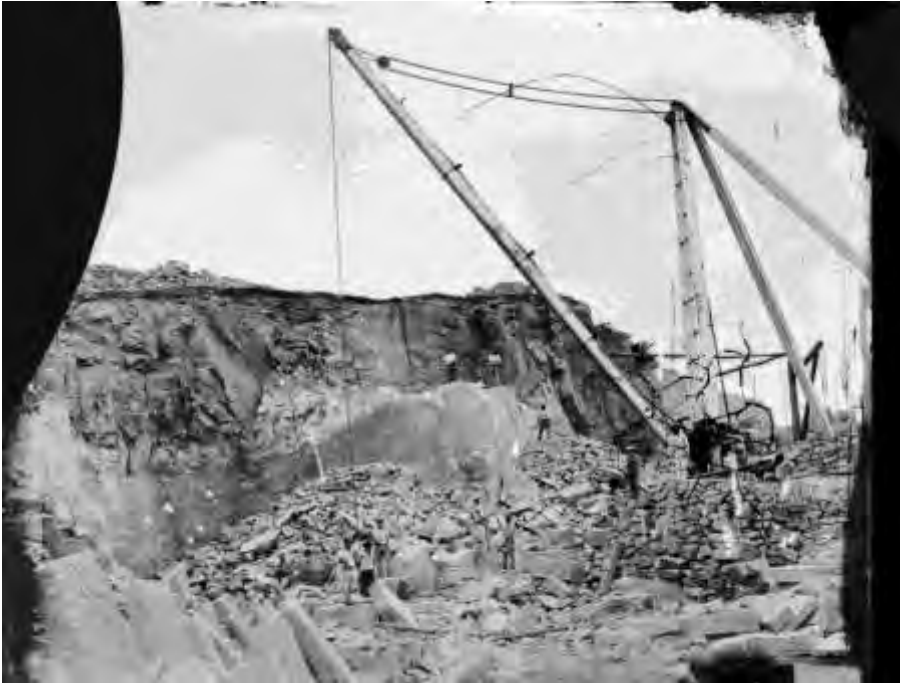
Figure 6 Neilson's patent five-ton derrick crane at Matson's quarry (Bald Hill Quarry) (Daintree, 1861)
